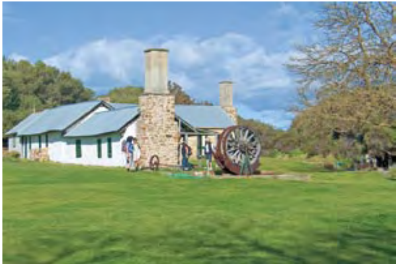
Ellensbrook Homestead. In the foreground are parts of the waterwheel that operated in the brook
